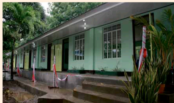
SHIMIZU’S six-classroom building at Venancio Trinidad Senior Memorial High School in Talisay, Batangas
